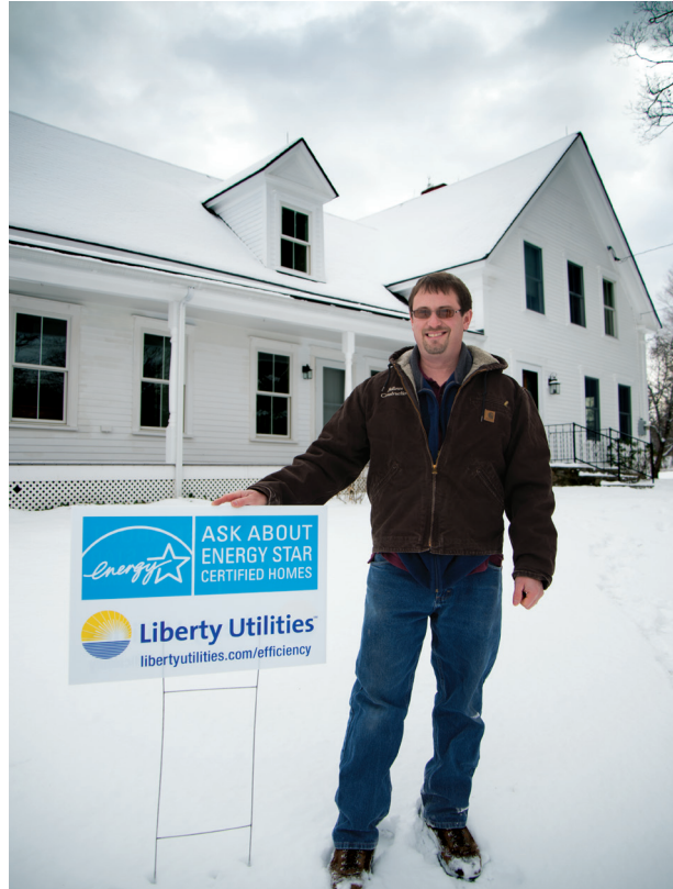
Barrett Bellows of Bellows Construction in front of a farmhouse originally built in the 1800's. After his extensive renovation, the home is now ENERGY STAR certified.
