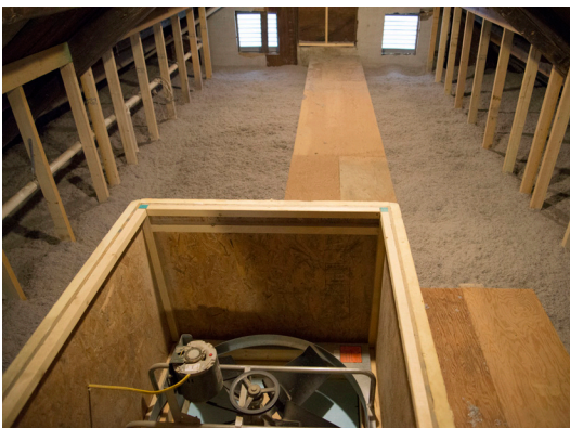
Attic space with whole-house fan that can be closed in winter. Loose fill insulation has an R-value of 55.
