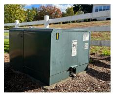
If your property has an underground electric service, you most likely have a box in your yard mounted on a cement or fiberglass pad. That box is called a transformer and it reduces the voltage coming from our distribution lines before entering your home.
