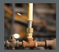
Corrugated stainless steel tubing (CSST) is a thin-walled metallic gas piping product that can be used as an alternative to conventional gas piping material. This flexible piping is commonly coated in a yellow plastic. If your home uses CSST, we recommend that it is inspected by a qualified plumber for proper installation and bonding. CSST that is not properly bonded could cause an accidental leak or fire when struck by lightning.
